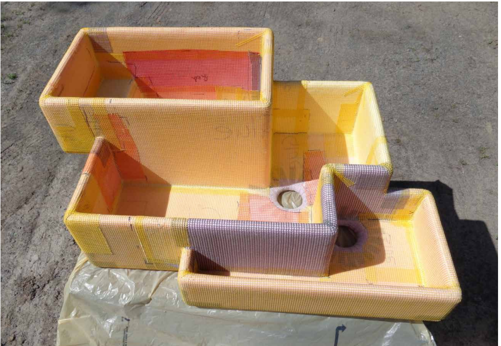
A complex trough completely wrapped in mesh.
