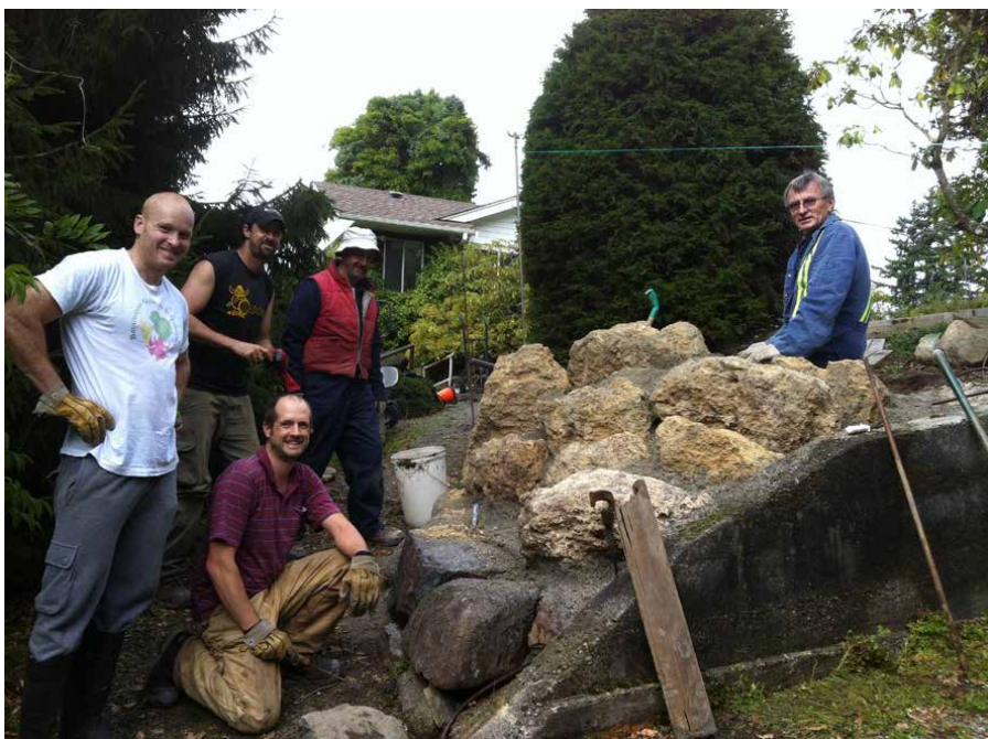
Building the tufa bed.
