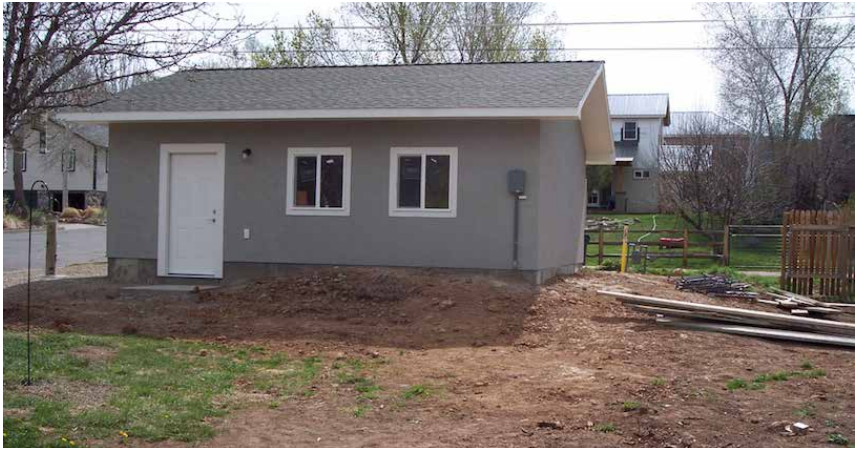
The new garage, with the pile of orange clay subsoil in front that would become Garage Hill.
